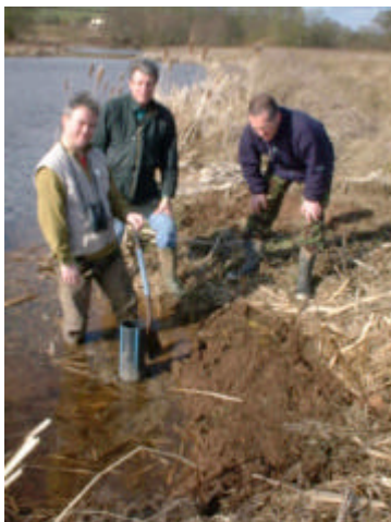
Joe, Tony, and Andy repairing the bund
